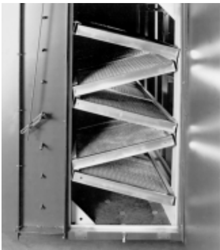
③ Optional inlet damper with V-bank filter
